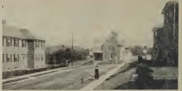
FIG. 9—NEWBURGH, N. Y.—STREET VIEW LUDLOW AND PEABODY, ARCHITECTS
